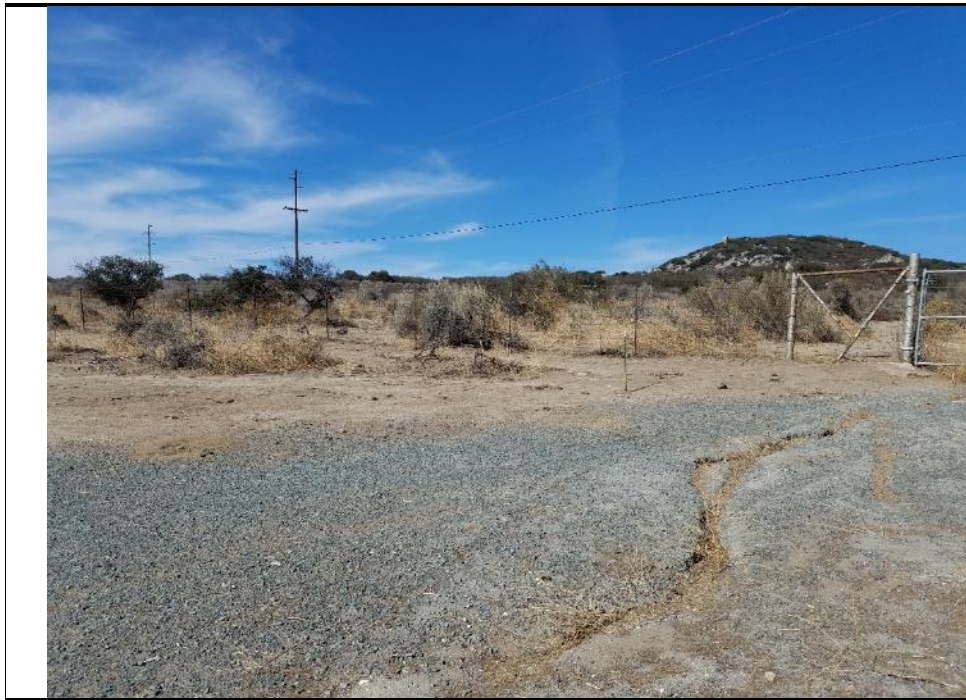
Photograph 4: Northwest-facing view of the western temporary access/entry/turn-around work area, as observed on November 15, 2018.
